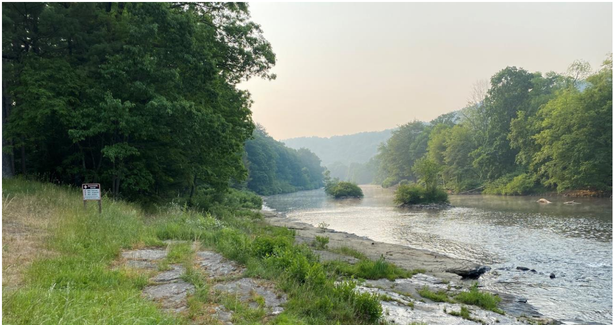
Figure 19: Below the failing dam, flat bedrock along the bank offers a scenic gathering location for families. The historical man-made islands were constructed of local mountain stone and sunken timber and made up the Susquehanna Boom, used to sort and control the flow of logs from 1851 to 1909.
