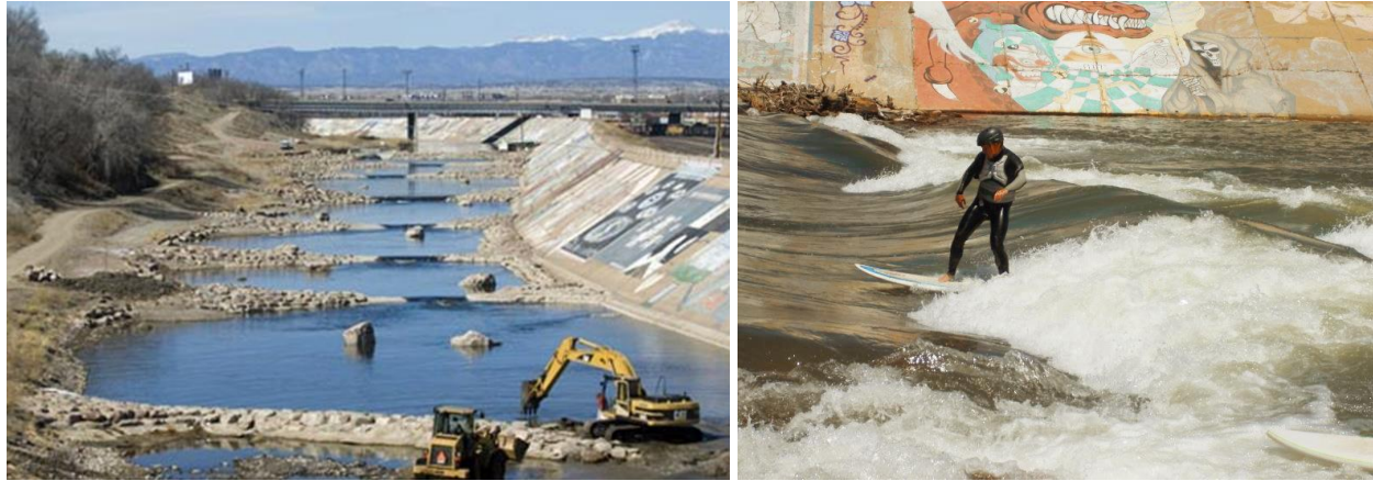
Figure 43: The West Branch of the Susquehanna widens in this section, spanning about 300 feet wide at Raftsmen Dam. The Pueblo, CO Whitewater Park, pictured under construction on the left (Bryan Kelsen, 2007) and in use at higher flows on the right, shows what multiple structures on a wide section of river can look like.
