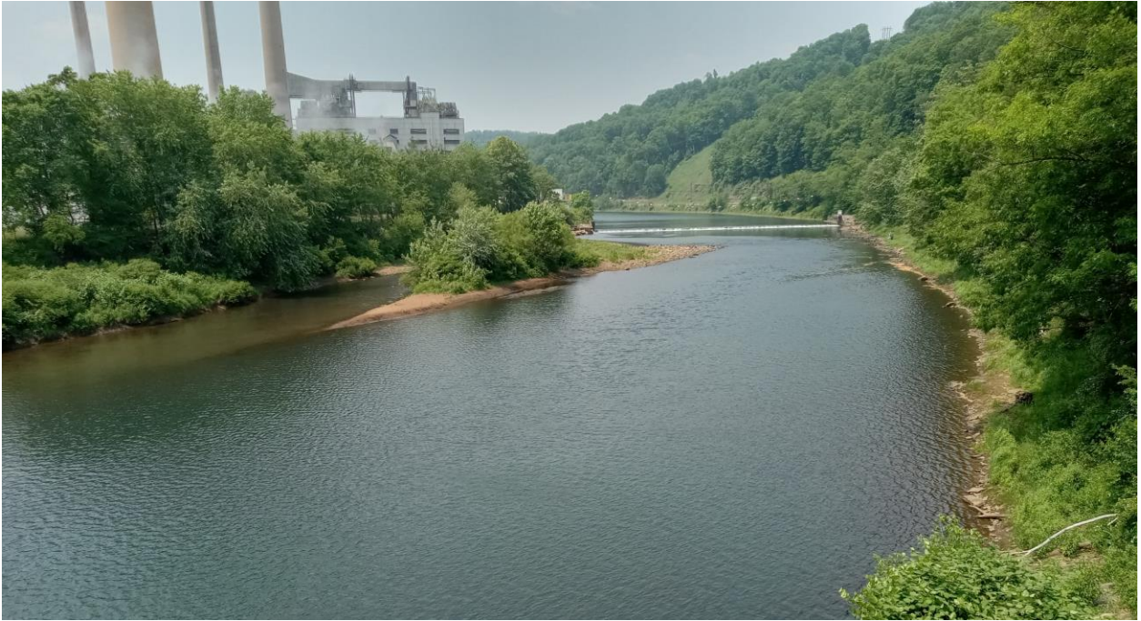
Figure 36: The Shawville Dam, owned by Gen On Energy, presents a dangerous and inconvenient portage. It is constrained by the power plant on river right and a steep embankment up to the highway on river left. Complete removal of this dam is recommended, for which a separate study is ongoing.
