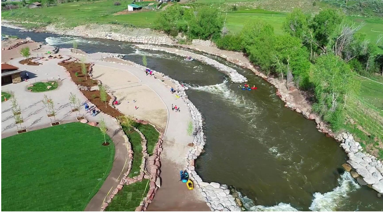
Figure 44: Riffle Bypass Feature at Eagle Whitewater Park.
