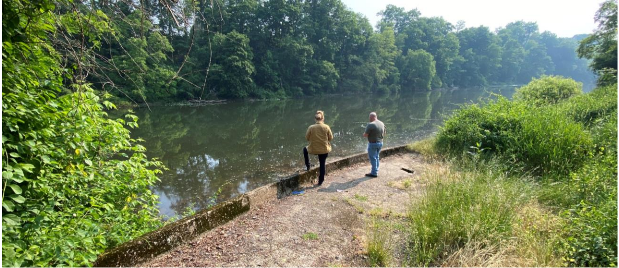
Figure 24: Concrete structure at Howe's Leather site that could be reconfigured to be a canoe/kayak launch or connected to trails at the planned camp ground. It is reported that this structure was a foundation from Susquehanna River's very first dam, created by "Irvin's Log Mill" to hold back logs as staging for the milling operation that was across river from the Anderson Creek Confluence. The concrete structure was later used for a raised steel tower/staircase that had a pedestrian suspension bridge tied into the hillside across the river, which was used by the factory workers at the mills and tanneries to walk from their homes to the factories.
