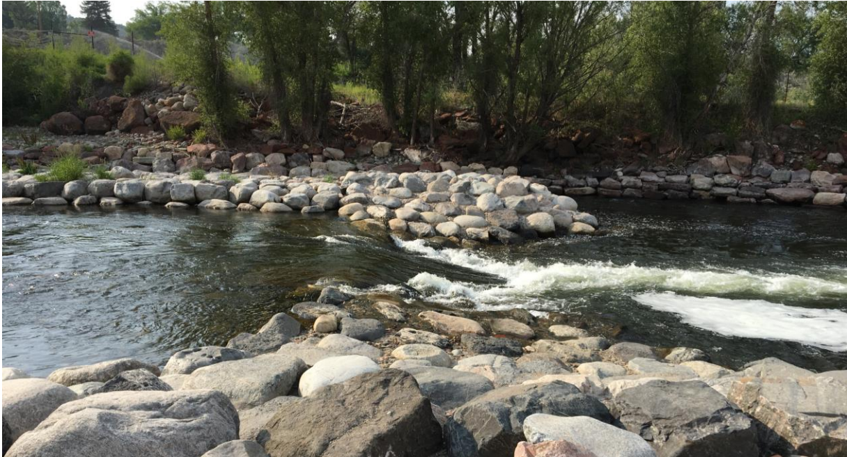
Figure 37: A similar Wave Feature at low flows in the S 2 O designed Eagle Whitewater Park
