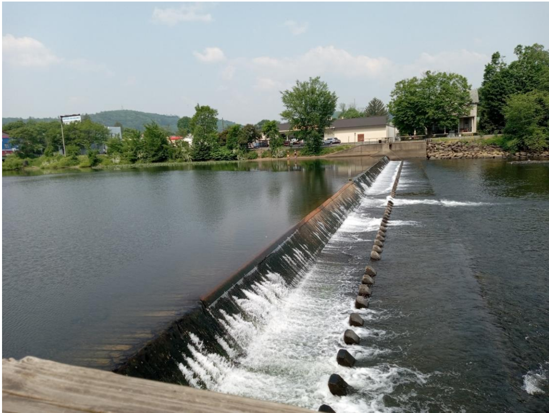
Figure 31: The Raftsman Dam is the subject of a conceptual design for removal and replacement with a whitewater structure. It is constructed of large timber framing, filled with rocks, and covered with wooden boards. A 60-foot section of the dam broke off in 2016, and the dam presents an ongoing maintenance issue for the Borough.
